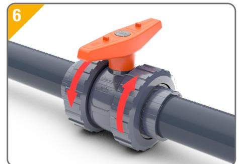
**6.** We put the valve back into the installation and tighten the nuts again.
